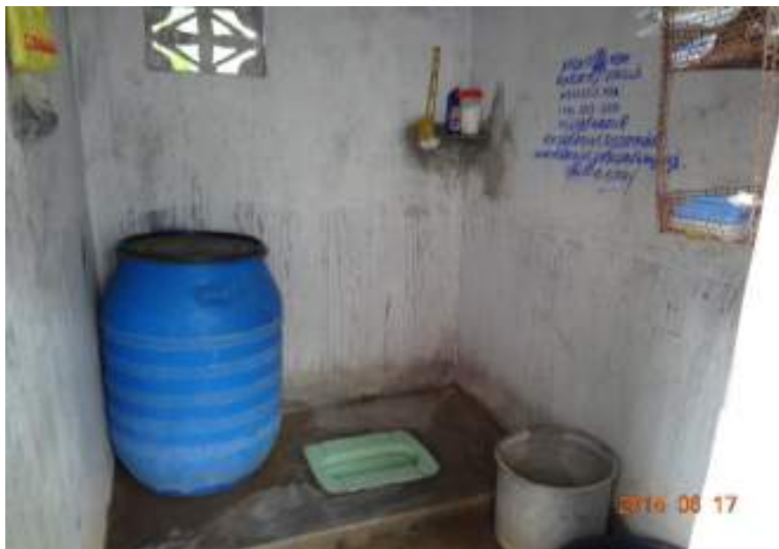
A toilet in Chaparathi Village built under the SBM
