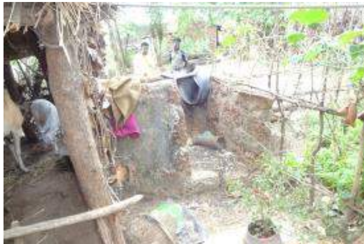
A defunct toilet with low walls
