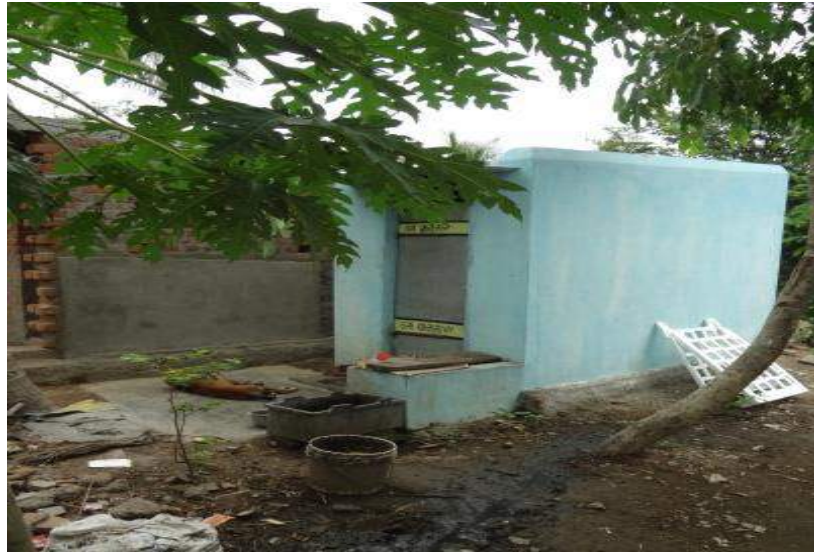
A Completed Toilet in Ganjam District
