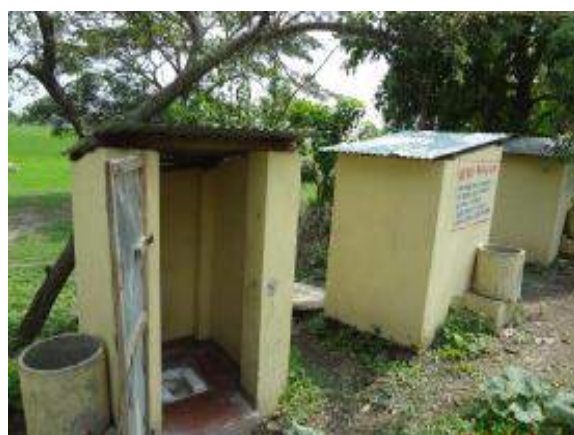
A completed toilet in Balasore District
